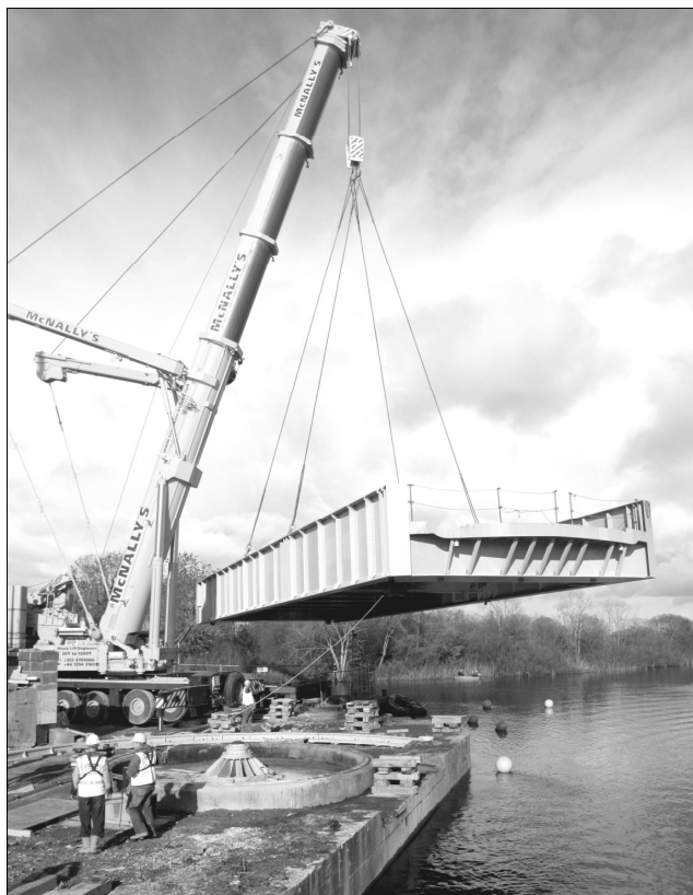
New swing section of Portumna bridge being lowered into position.
